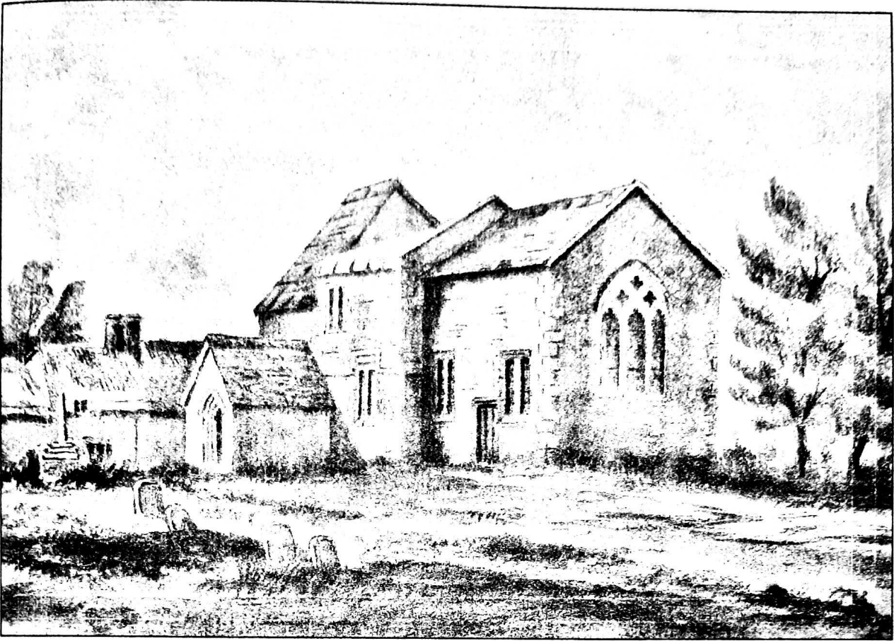
St Mary's Church, Cottisford, south east view in 1825 (J.C. Blomfield).
